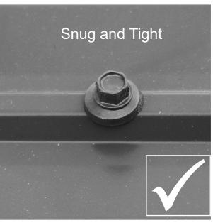
The roofing screws can easily crush the Roof Panels and Roof Edges when using a power drill. We recommend hand tightening the roofing screws so that they sit snug and tight to the roofing material.
